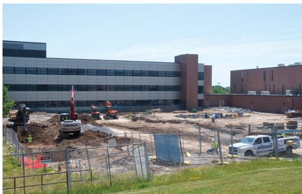
Construction of the new facility began over the summer.
