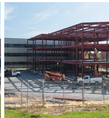
The building connects to Golisano College of Computing and Information Sciences.
