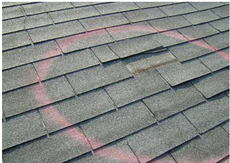
Rooftop Damage: RIT researchers are looking to automatically quantify the amount of damage to rooftops caused by hail (top) and wind (bottom) to help property casualty insurance inspectors carry out their inspections in a faster and more accurate fashion to settle claims for their clients.
